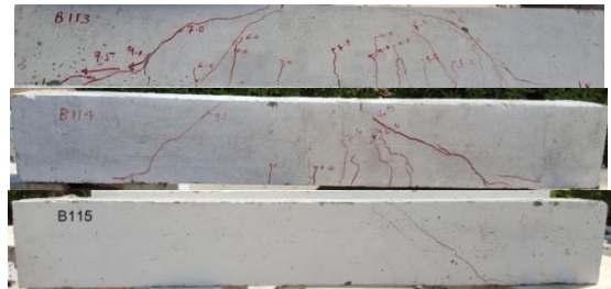
Figure 6. Crack pattern of group two ferroccement beams
