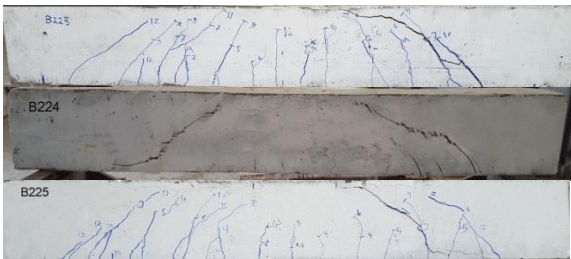
Figure 8. Crack pattern of group four ferroccement beams
