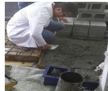
Figure 5: Practical Steps to Grinded Surface
