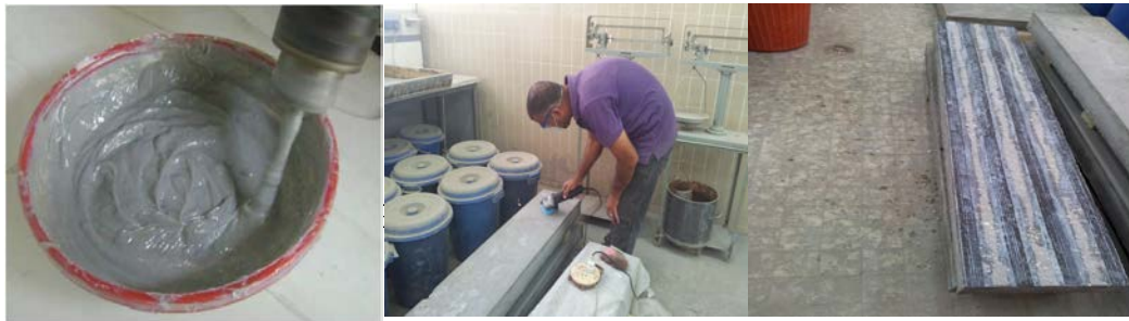
Fig. (3): Preparing and application of CFRP strips
