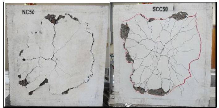
Figure (14) - Crack pattern of SCC and NC slabs failed in punching shear
