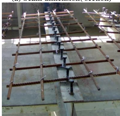
(b) Section, studs and reinforcement
