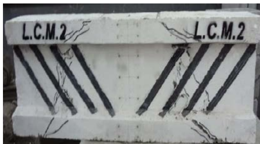
Fig. (4): Shear cracks pattern of L.C.M.2 beam.
