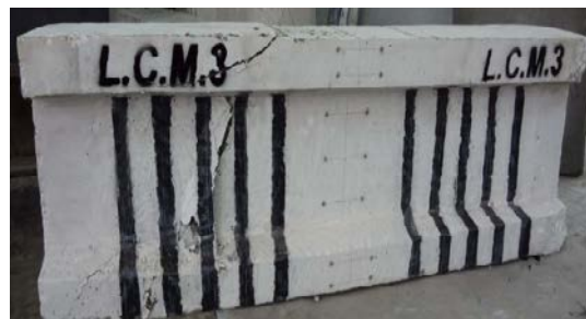
Fig(5): Shear cracks pattern of L.C.M.3 beam.
