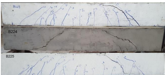
Figure 8. Crack pattern of group four ferroccement beams
