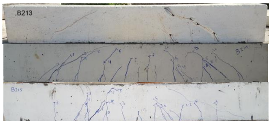
Figure 7. Crack pattern of group three ferroccement beams
