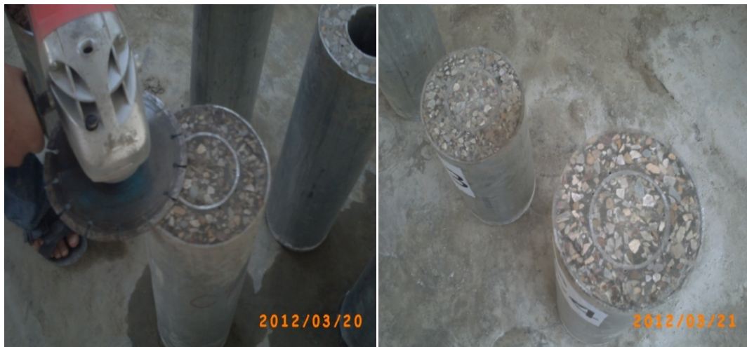
Fig. (3) :Smoothing the columns surface
