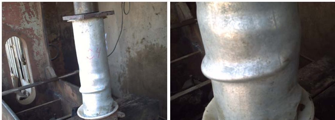
Fig. (16): Failure Pattern of Sample C4
