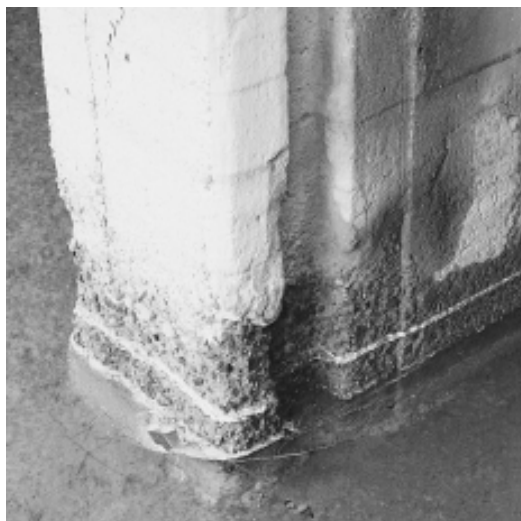
Fig.(1). Deterioration of concrete by sulfate solution
