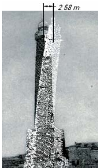
Figure 10. Estimated leaning during the last 90 years.
