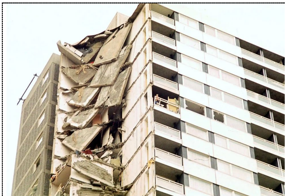
Fig. 2: The collapse of Ronan Point, 1968 [31].
