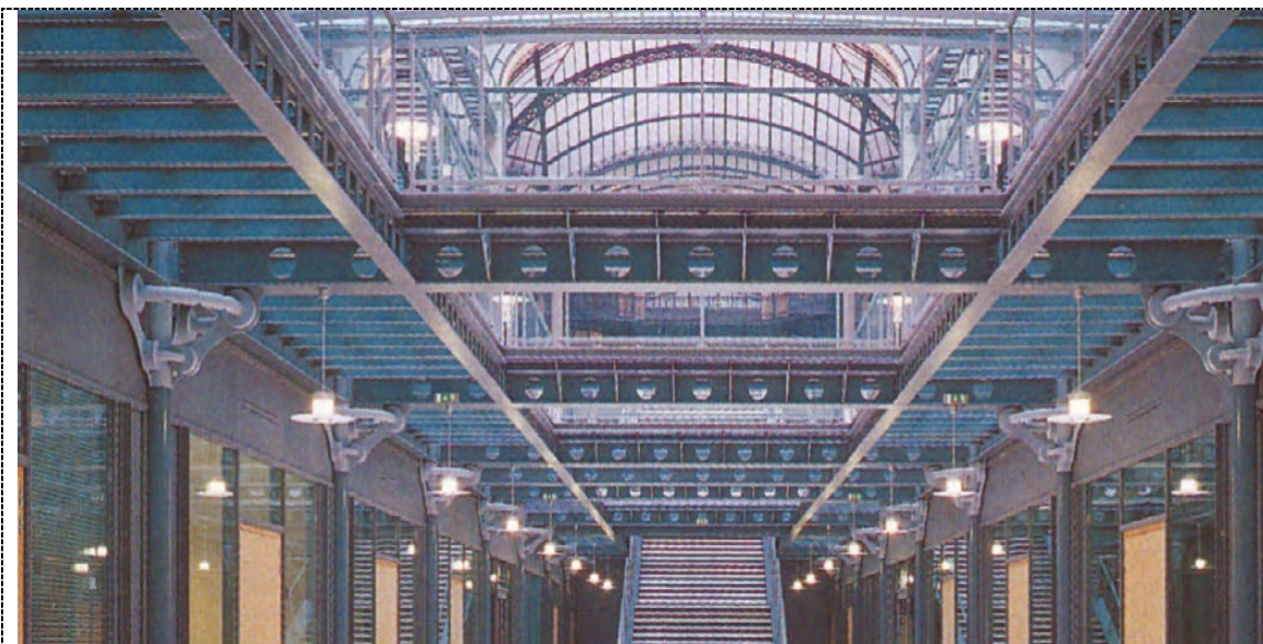
Fig. 1: Renovation using perforated beams at the headquarters of Crédit Lyonnais, Paris [6].
