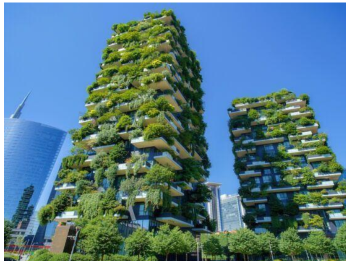
Fig. 2: The external facades of the Bosco Verticale towers, Milan [5].
